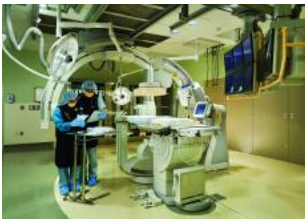
Suspended equipment keeps rooms free of obstacles like electrical cords and oxygen lines.
